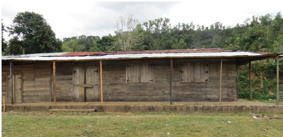
The school at Ambohimanarina with a (mostly) new roof
