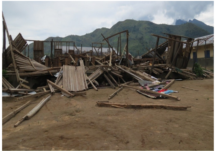
School in the village of Mandena after cyclone Enawo
