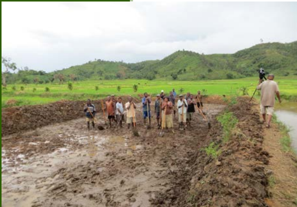
Members of a village association working on constructing a fish pond for fony
