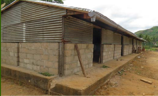
Mandena village school with repairs almost finished
